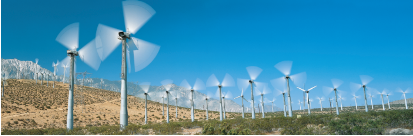
Figure 3 The spinning blades of a wind turbine are connected to a generator. When winds cause the blades to spin faster, the generator produces more energy.
