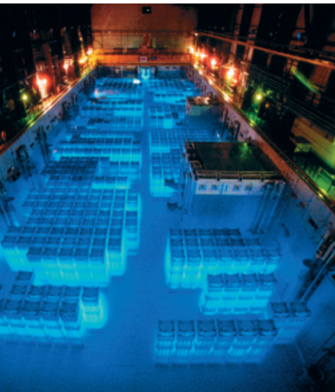
Figure 6 These water pools store radioactive wastes. The blue glow indicates that the waste products are highly radioactive.
